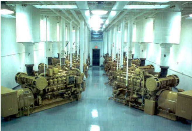
Figure 15. Eight 800-kW Caterpillar engines supply power to a plastics plant in Illinois. Design and photo by LaSalle Associates.
