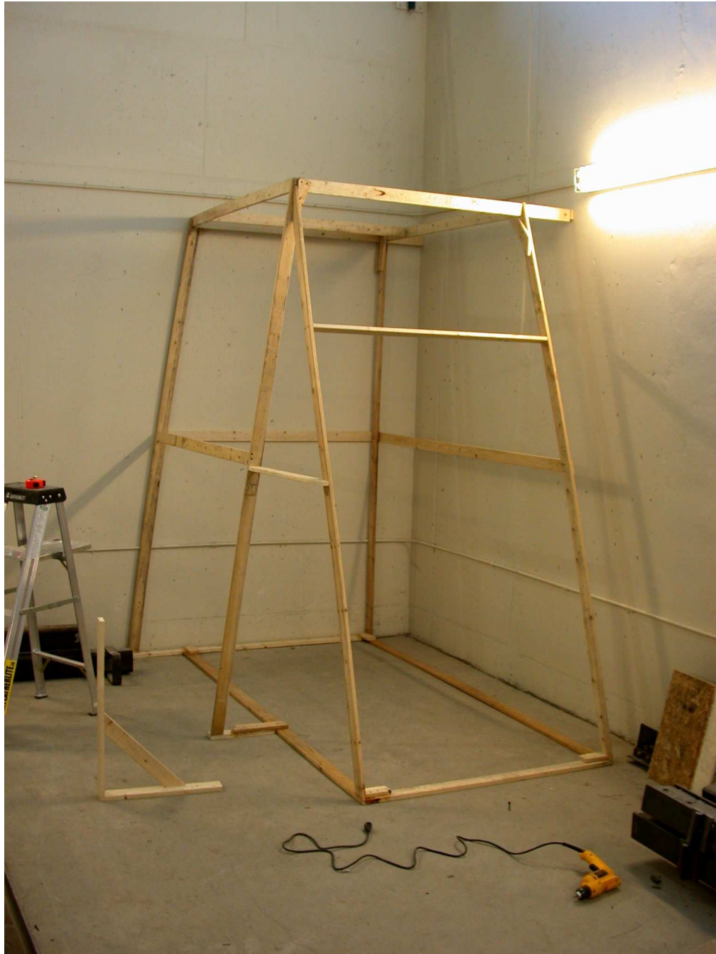
Figure B.5: Tower support structure
