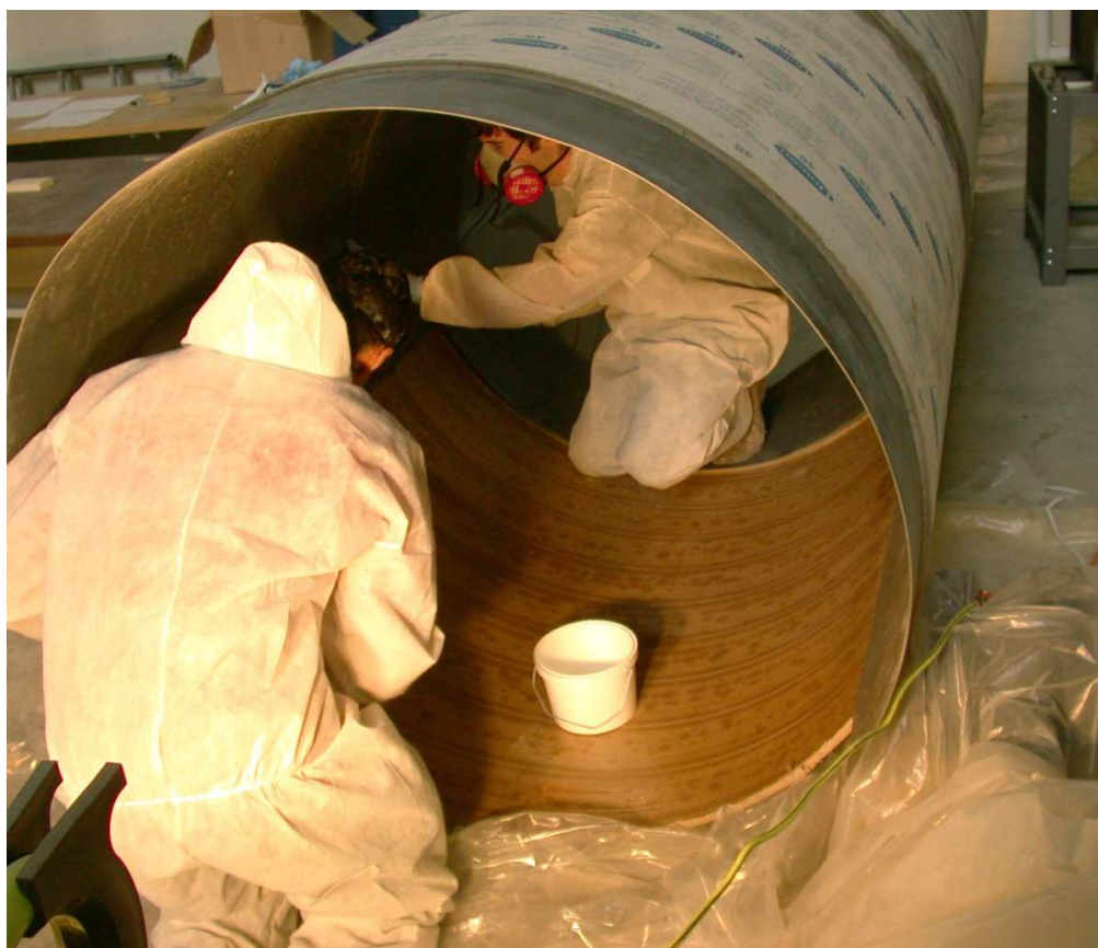
Figure B.3: Lining the inside of the Sonotubes with PVC sheets.
